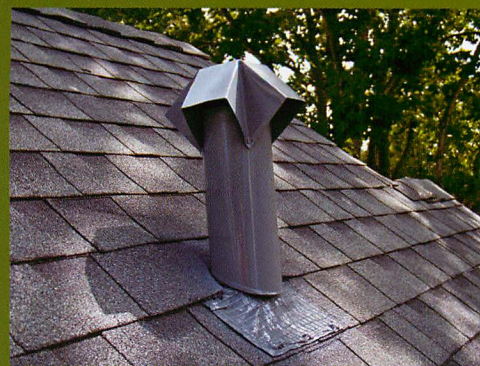
SquirrelGard™ Installed on roof.
